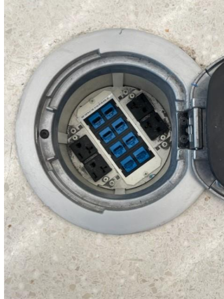
Interior of one of the floor outlets
